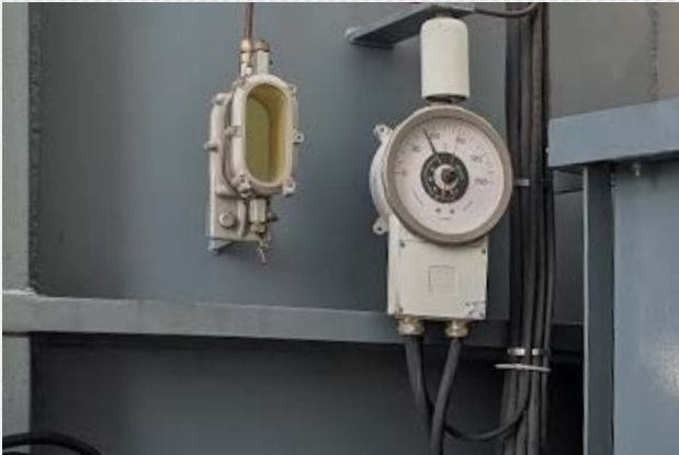
Figure 5. The measurement position behind the reactor pressure indicator.
